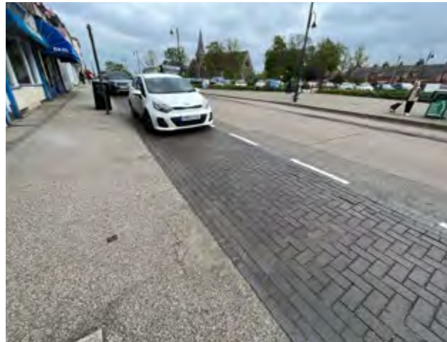
Figure 34: High quality materials distinguish the parking bays.
