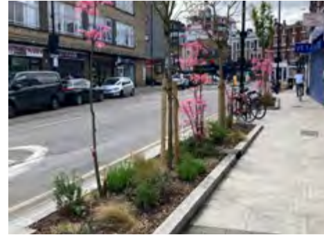
High Street rain garden - linear rain garden for surface water mitigation
