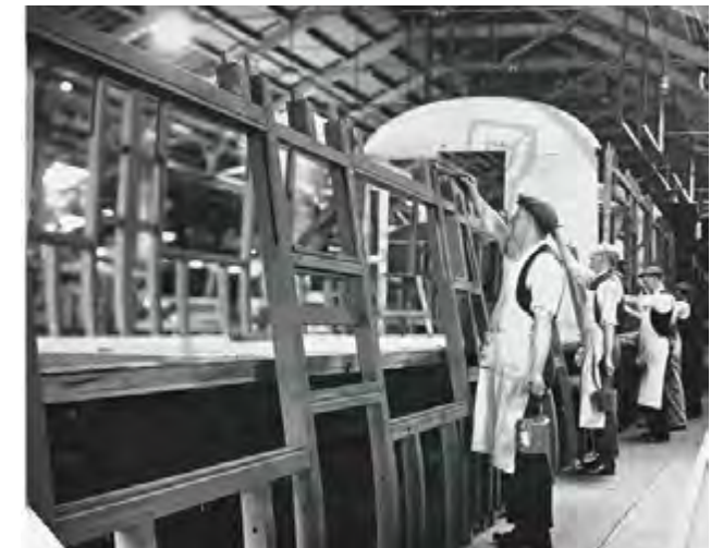
Figure 05: The Wolverton Railway Works Paint Shop.
