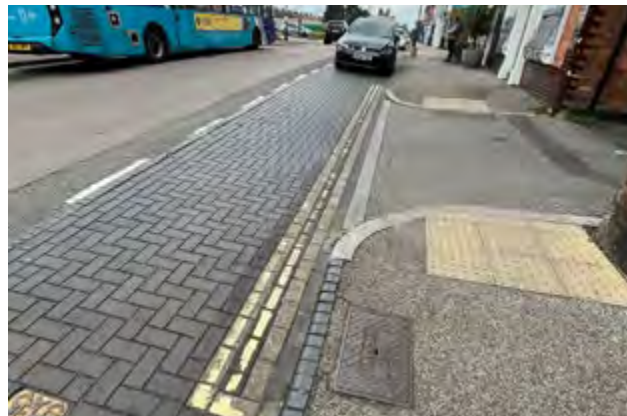
Figure 20: An example of tactile paving in the site area.
