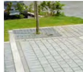
Edge kerb to ramps and 'blended crossing' - Granite Conservation edging kerb. Laid flush. Colour: Silver / Grey.
