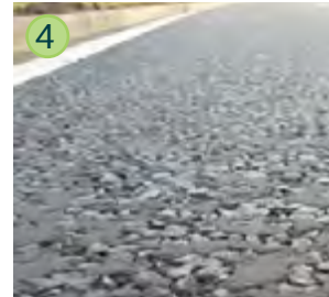
Carriageway, raised table (western roundabout), ramps to pedestrian crossing points & vehicular approaches to blended crossings - Hot-rolled asphalt surfacing with pre-coated chipping rolled in. Colour: Black.
