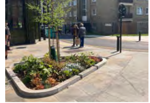
Rain garden - corner shaped rain garden for surface water mitigation
