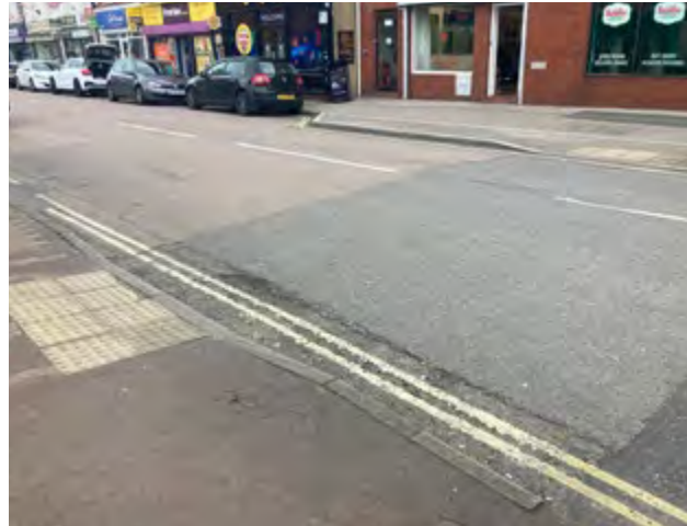
Figure 18: Dropped kerb and tactile paving informal crossing across Church Street.
