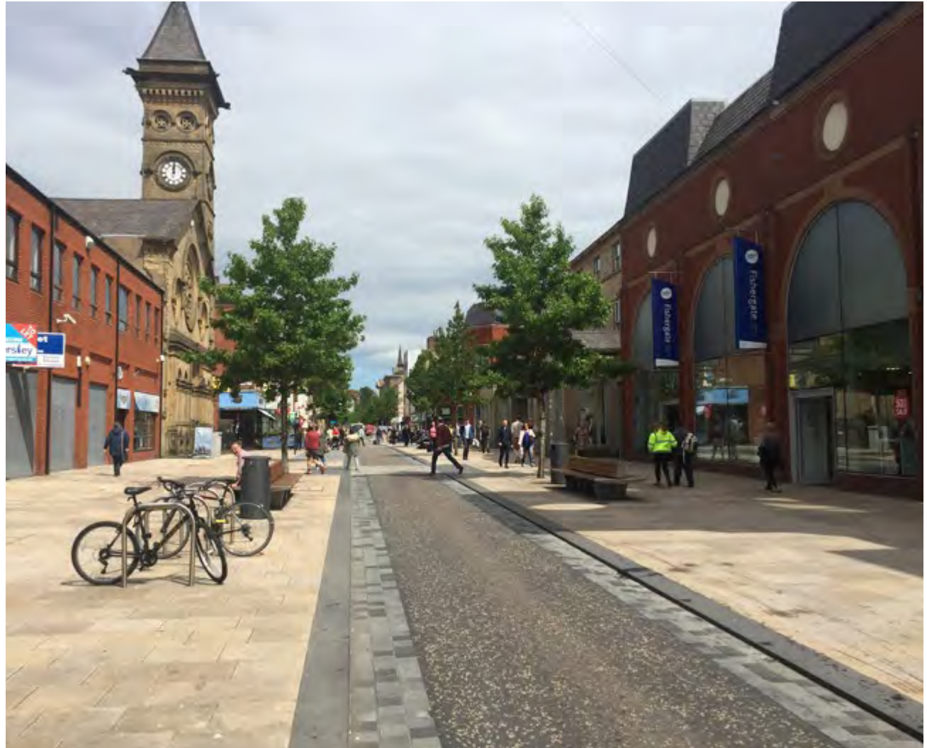
Figure 66: A south westerly view along Church Street, Preston showing the carriageway and pedestrian areas in different surfacing.
