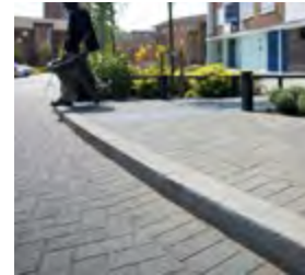
Kerbs to carriageway & parking bays - Granite Conservation kerb. Laid with 100mm upstand. Colour: Silver / Grey.
